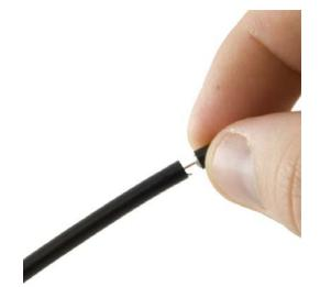
Pull wire out of cable stripper and remove remnants from first cut revealing center conductor.
