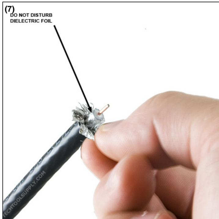
7. Now you will be folding the cables first three layers of shielding back out of the way. The best way to fold back the multiple layers of shielding is with your finger tips or a small flat tool. Careful not to push too hard with your fingertips; the cables braid can prick your finger tips.
